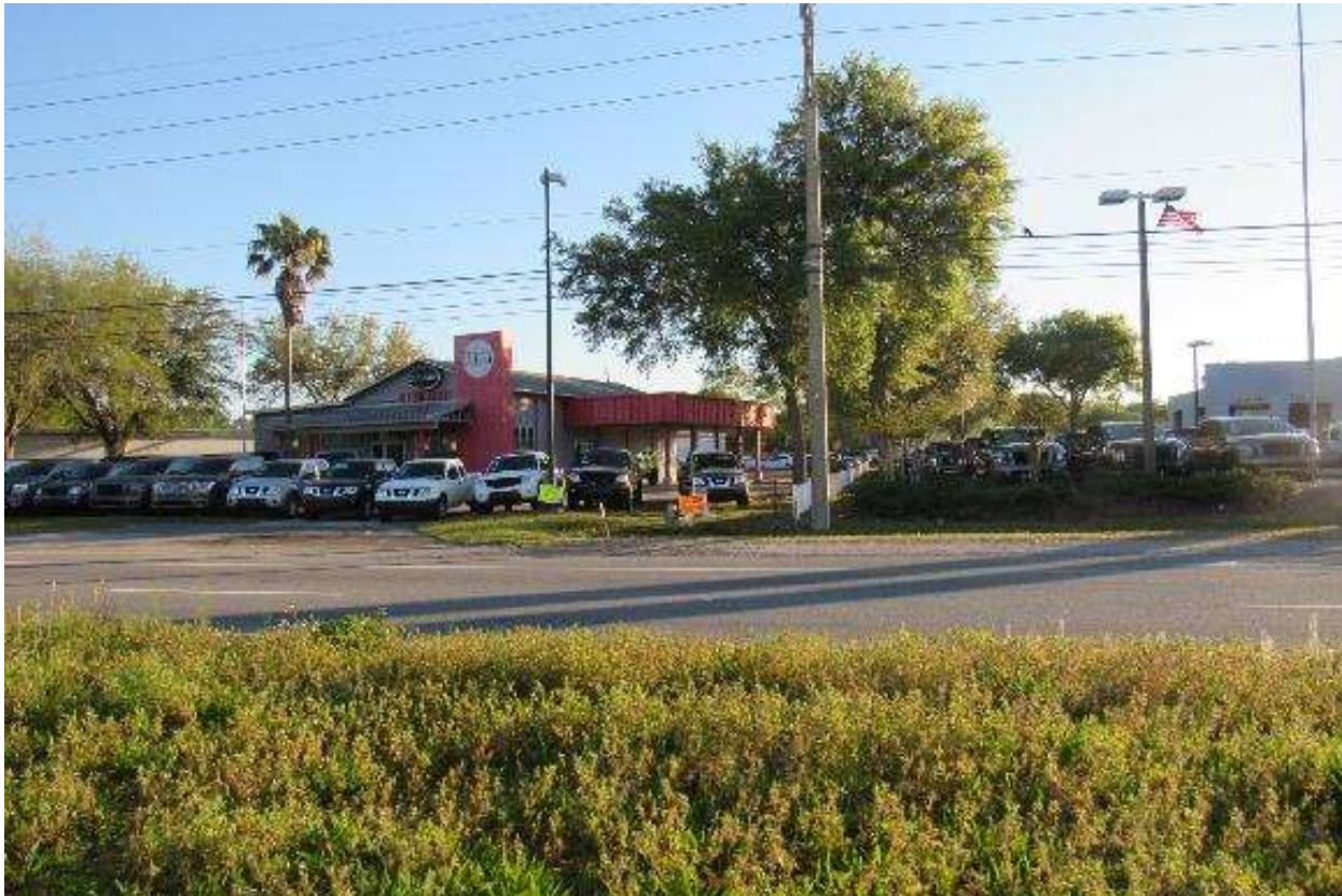
View of subject site.
